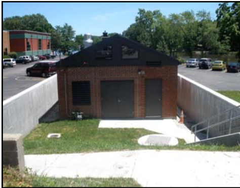
This pump station in Ottawa, IL is an example of VSA's numerous municipal projects.
