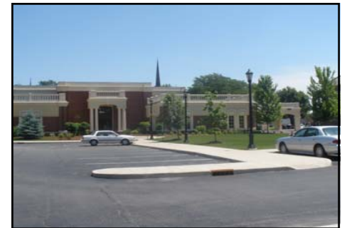
VSA created the site development plan for this new facility in Ottawa, IL.
